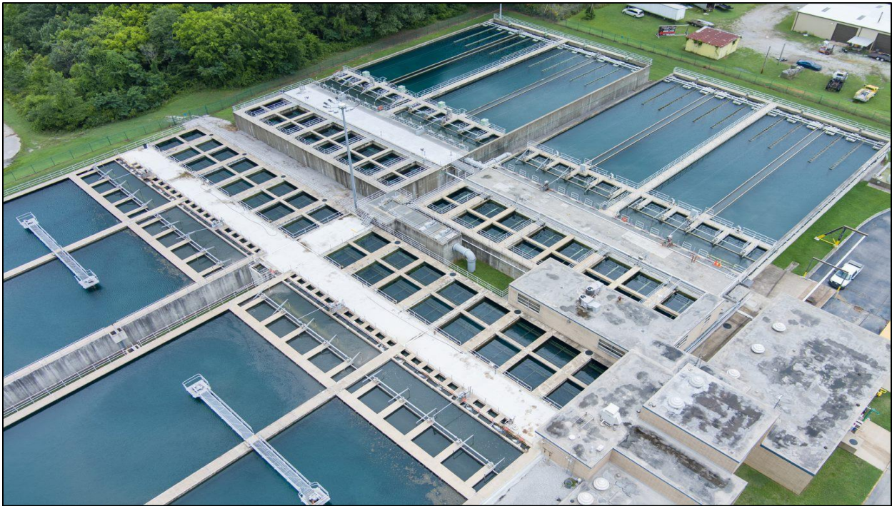
The two photos above show the South Parkway Water Treatment Plant, one of three Huntsville Utilities facilities that treat water taken directly from the Tennessee River. Over the next four years, nearly $23 million will be spent to rehab this facility which has been in service since 1964. The project is being funded through low interest Alabama State Revolving Fund (SRF) loans and is expected to be complete in 2025.
