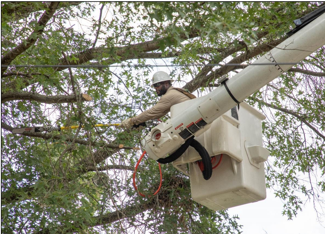
A major expense each year for the Electric department is line clearance or keeping power lines free of obstructions.
